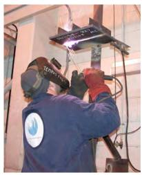
they undertake in Portland Harbour. A WPS was developed and welder testing carried out to ISO 15614-1 and 287-1 on high strength steel, using basic low hydrogen electrodes with welding being carried out in the overhead position. **Holstan**, who specialise in pressure pipework systems for the heating industry asked us to
