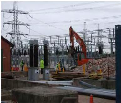
provide on-site aluminium MIG training for the substation power distribution work they undertake. Welders are involved with replacing old copper workings and the old concrete pylons with aluminium. The photo above shows the site at Capenhurst under major reconstruction.
