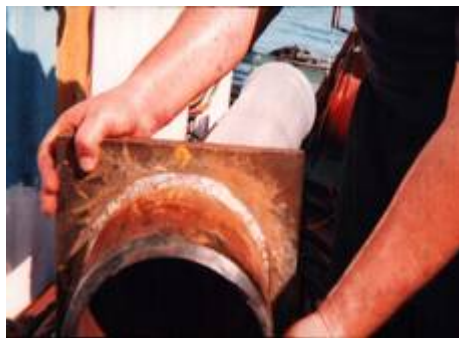
Photo shows the test sample weld.
