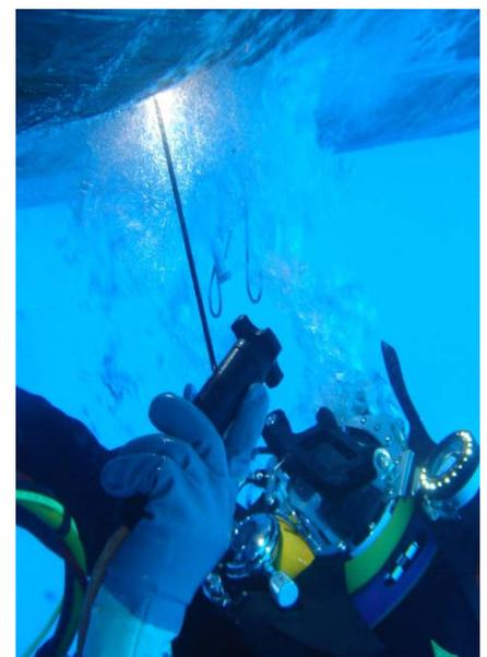
consisted of repairing a number of cracks in the underside of the hull using our **Barracuda Gold** welding
