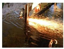
This invloved cutting approx 12m of trench piling in shallow water (2-4ft) on vertical bracings. This was carried out in order to return the river to its natural levels to help encourage wild life. We are pleased to report Swordfish electrode, keeps finding new niche markets around the world, with more and more orders for this product for both above and below the waterline. This electrode offers great alternative to traditional exothermic/oxy-arc cutting
