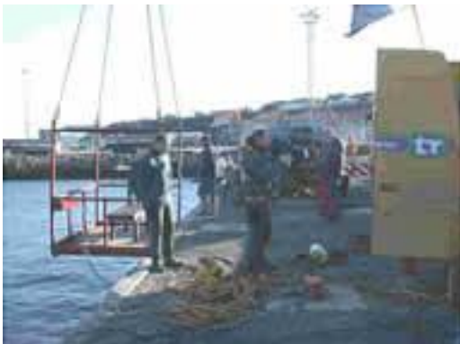
On site at Co Wexford harbour in Ireland
